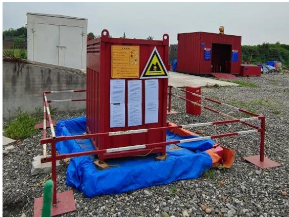
钻井期间危废暂存箱及防溢托盘
